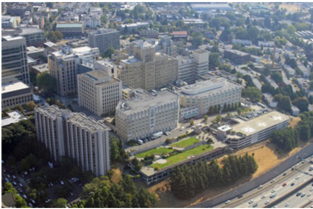
Figure 1 Aerial photo of the current Harborview Medical Center campus, Seattle, Washington.
